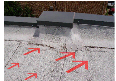
note alegstoring and deteriorated flashing
