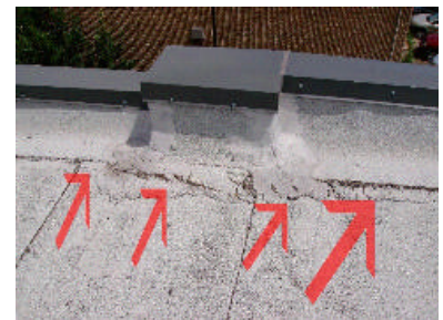
note alegstoring and deteriorated flashing
