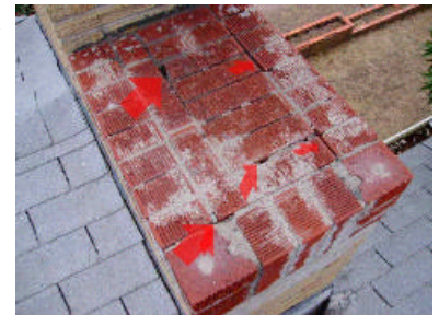
small crack in rain cap
